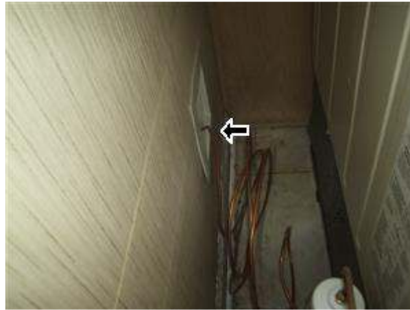
4.2 Picture 2 water supply to ice maker
