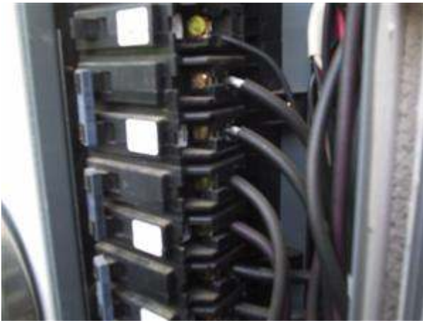
2.2 Picture 1 main panel
