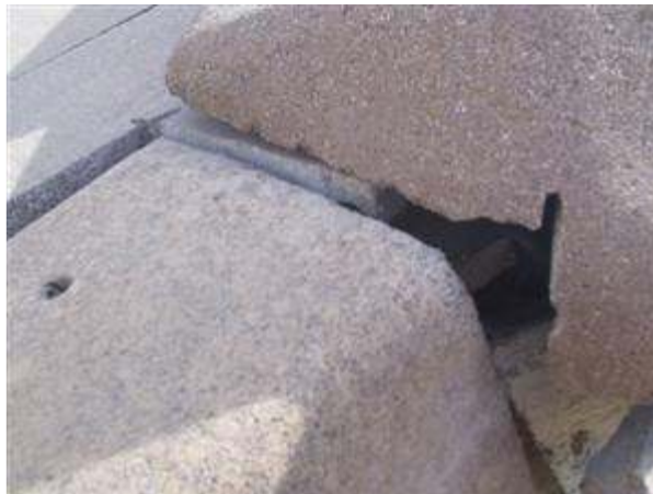
5.0 Picture 2 exposed roof sheathing
