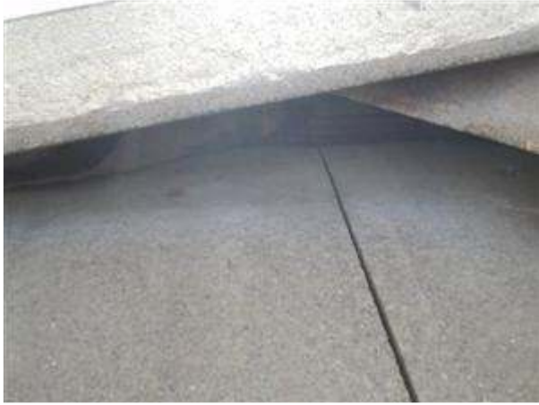
5.0 Picture 5 loosely fitted ridge cap
