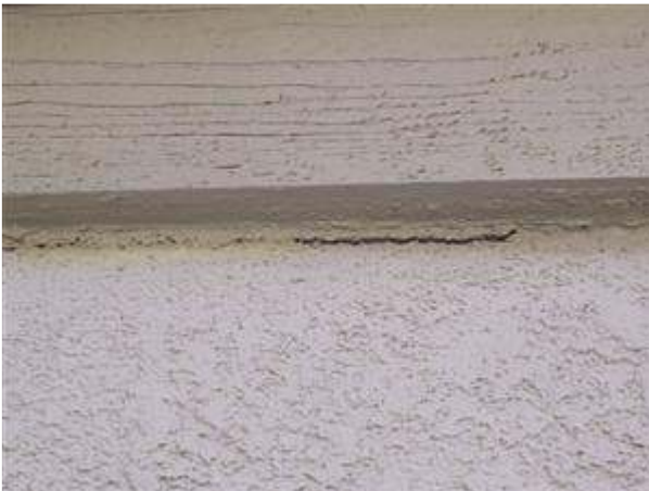
1.0 Picture 1 trim at back of garage
