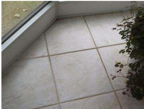
9.2 Picture 2 patio floor
