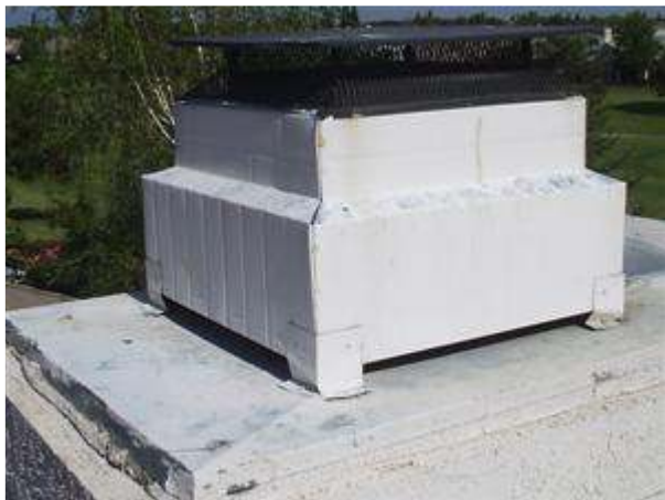
11.0 Picture 1 chimney cap
