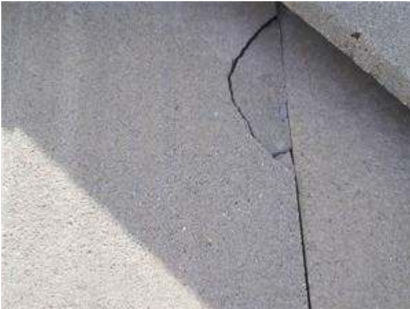
5.0 Picture 1 cracked tile
