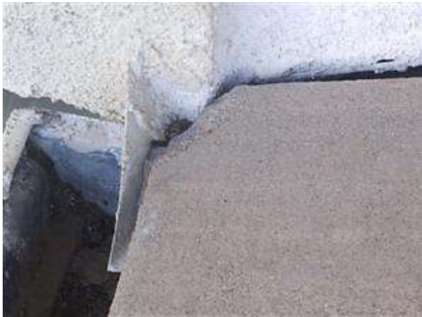
5.1 Picture 1 kick out flashing
